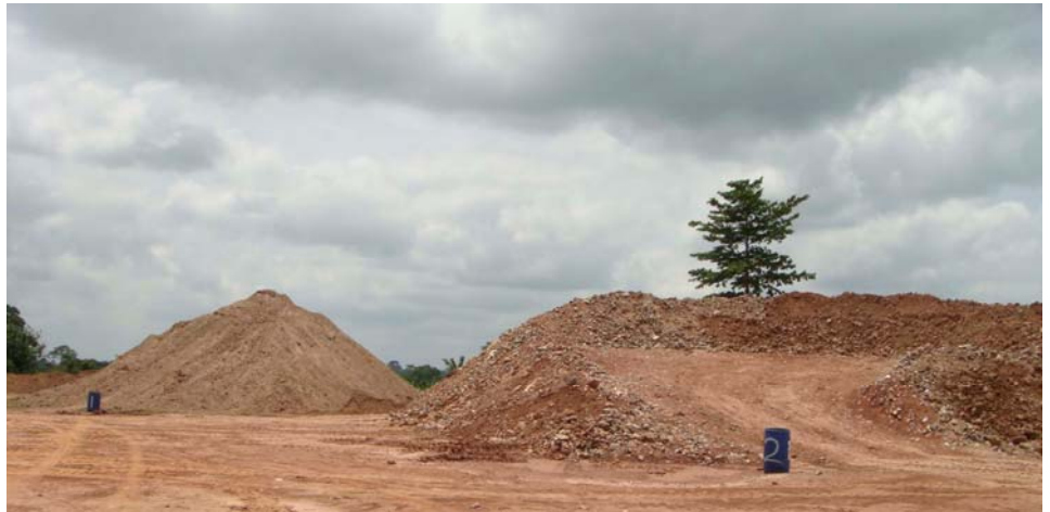
Stockpiles 1 and 2 on the ROM pad
