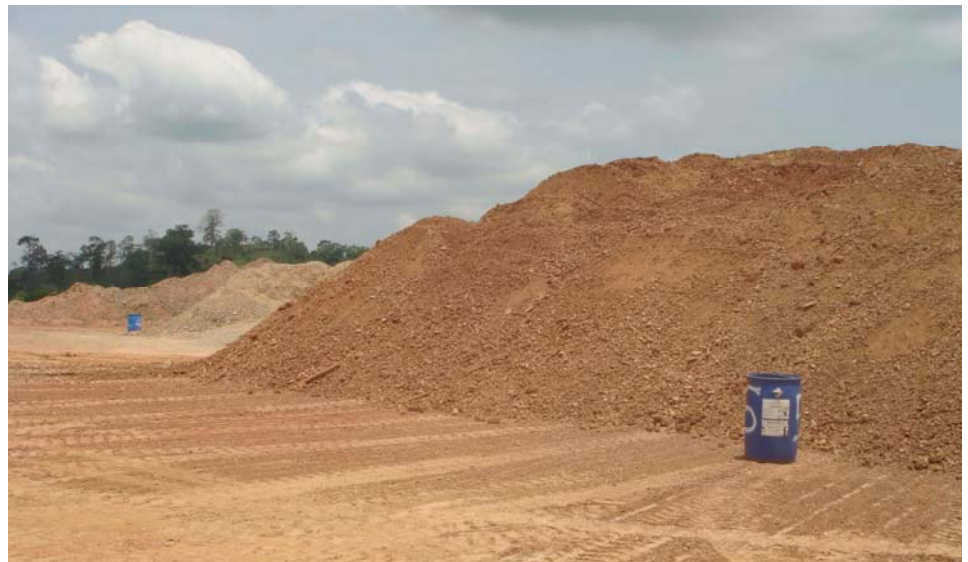
Stockpiles 4 and 5 on the ROM pad
