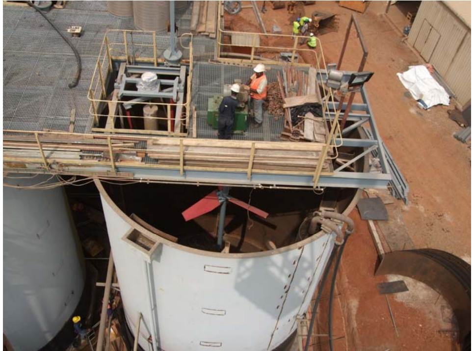
Refitting of motors to adsorption tank agitators.
