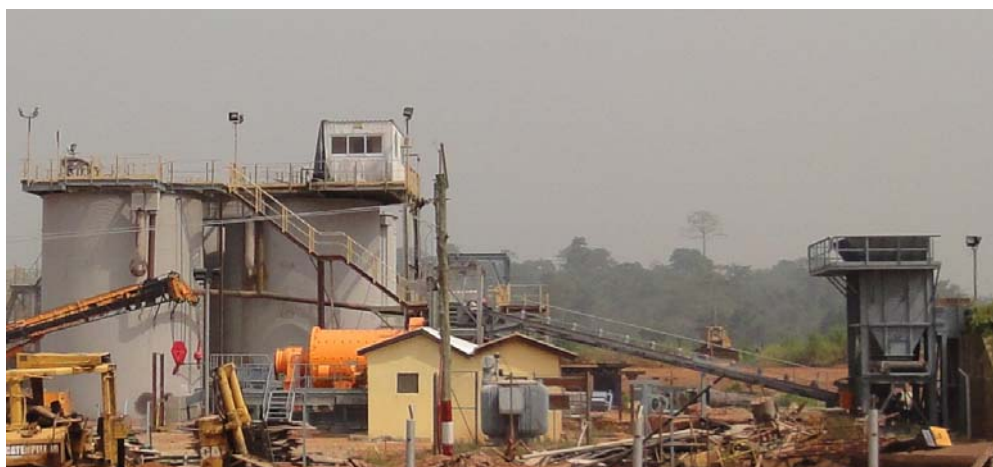
Refurbished ore handling system and ball mill awaiting final testing.
