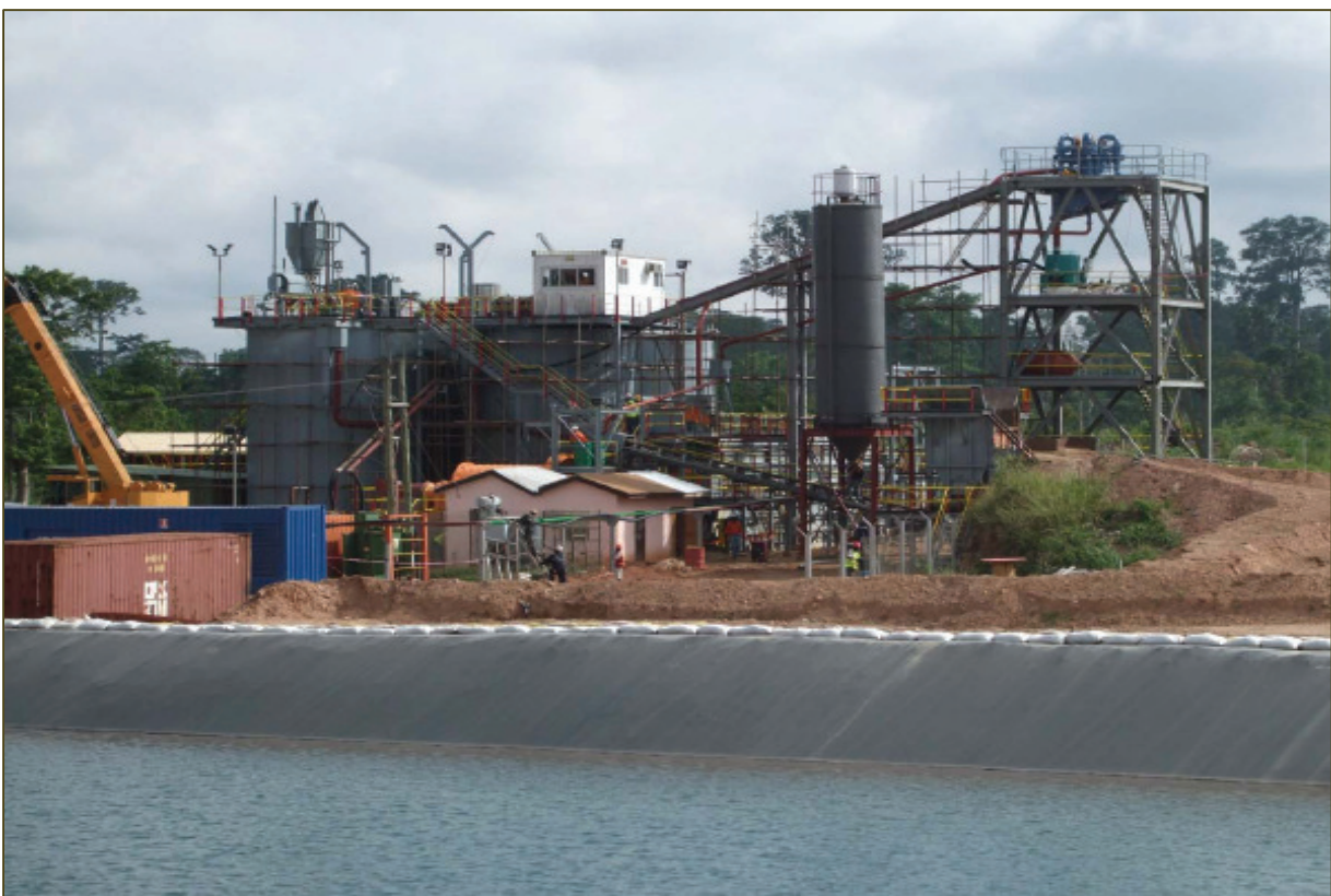
Picture 1 : CIL (Carbon In Leach) Plant in Operation at Konongo Gold Project
